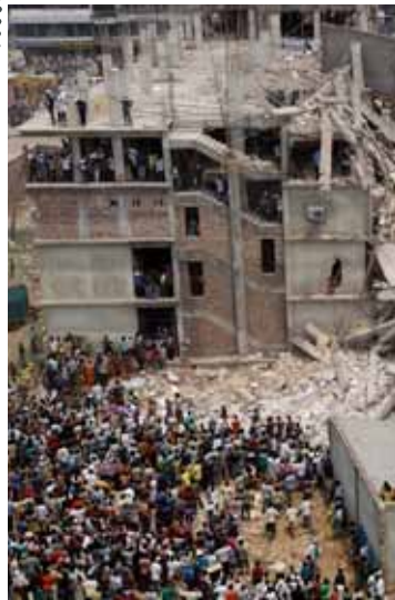
Dhaka Savar Building Collapse: rijans [flickr.com/photos/rijans]
